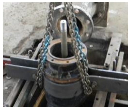
Figure 5 – Bowl Resting on Support Beams
