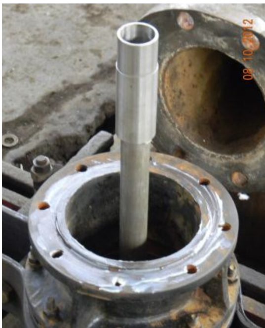
Figure 7 – Mounting Threaded Coupling on shaft and applying Grease over flange faces
