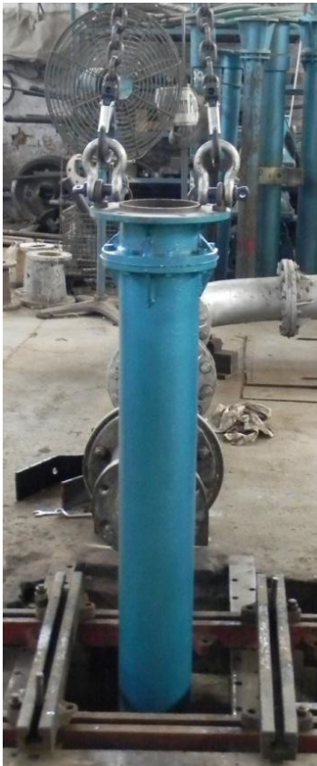
Figure 14 – Lowering the entire assembly
